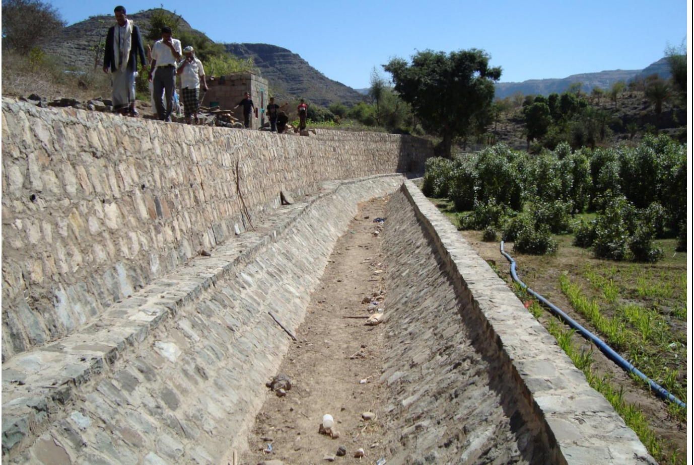
LINED PORTION OF CANAL
