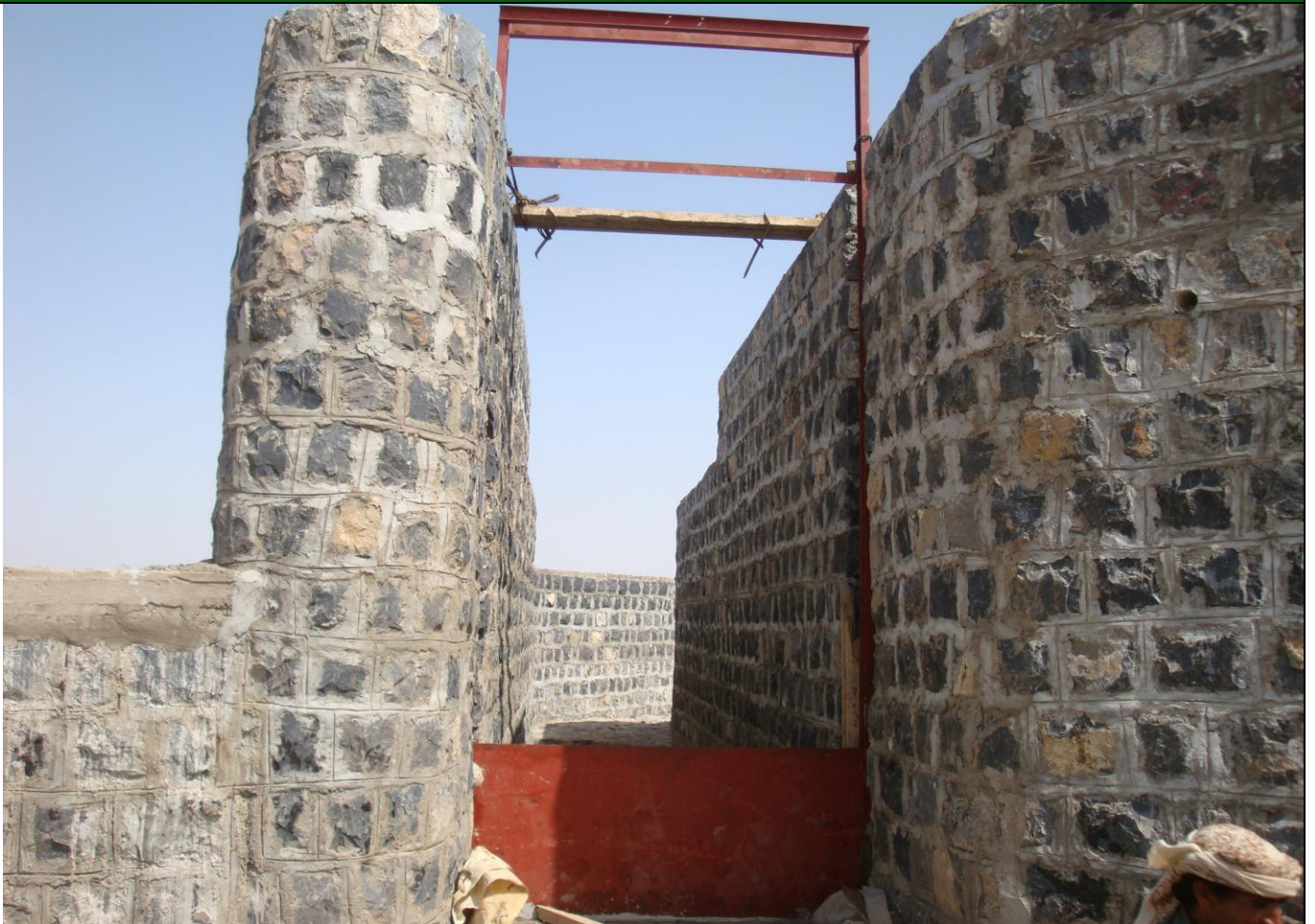
DOWNSTREAM VIEW OF THE WEIR, AND SILT SLUICE
