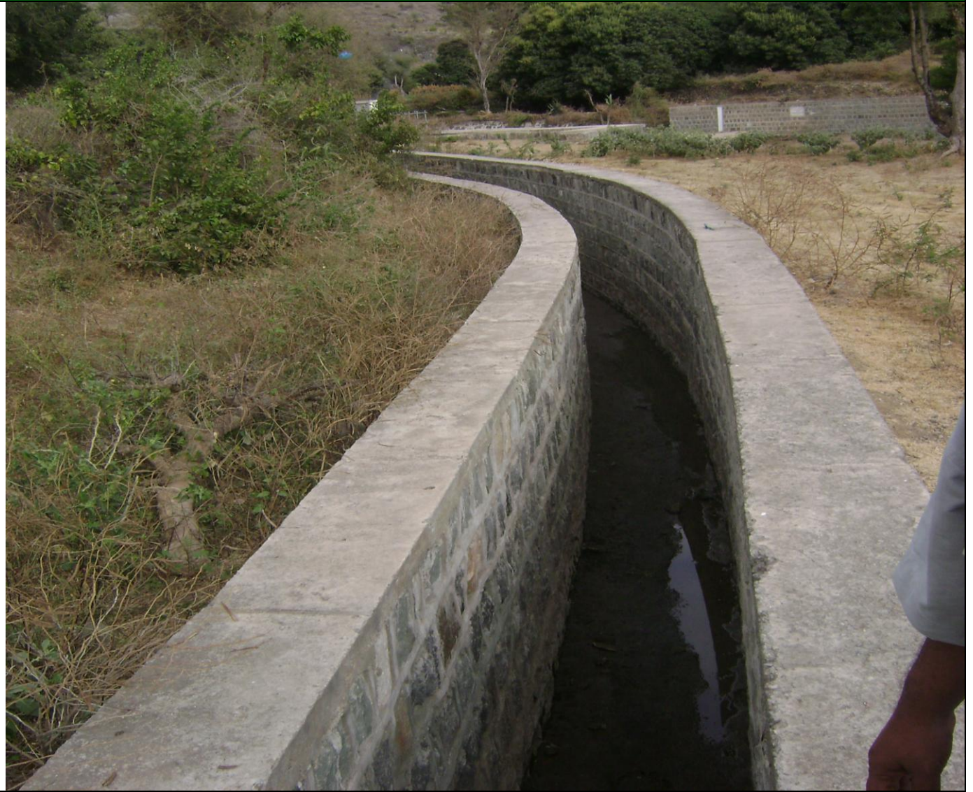
CANAL HAVING BOTH SIDES AS MASONRY WALL
