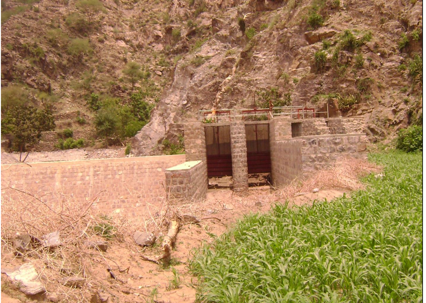
DOWNSTREAM VIEW OF THE SILT SLUICES AND PART CANAL INTAKE
