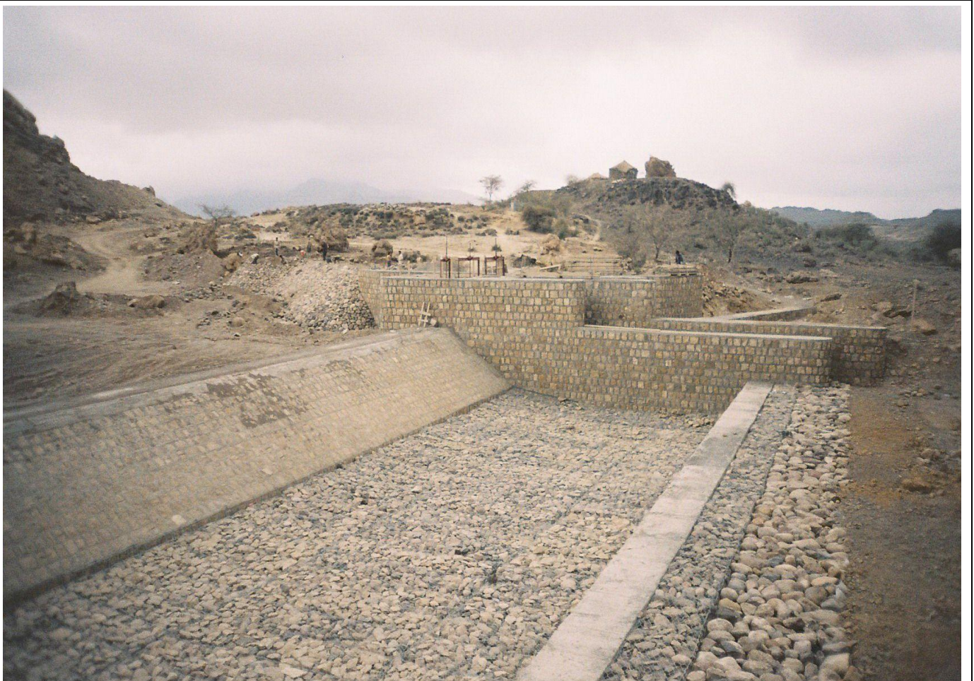
CANAL INTAKES AND SILT SLUICE VIEW FROM UPSTREAM
