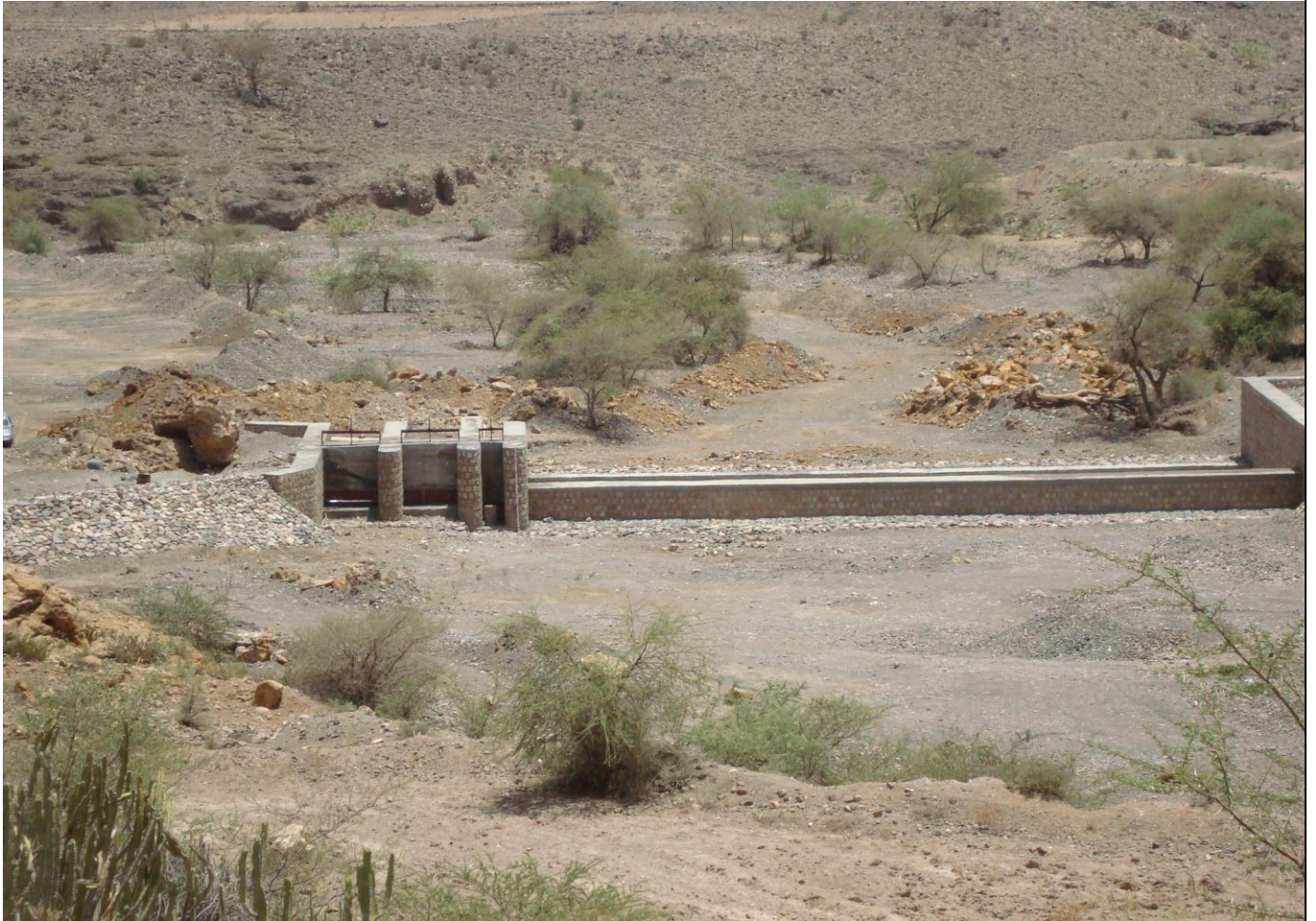
SPATE DIVERSION WORKS VIEW FROM UPSTREAM
