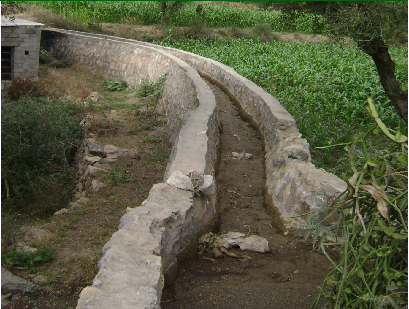
CANAL IN MASONRY AQUEDUCT
