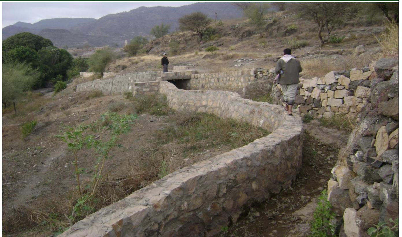
CANAL HAVING ONE SIDE AS MASONRY WALL
